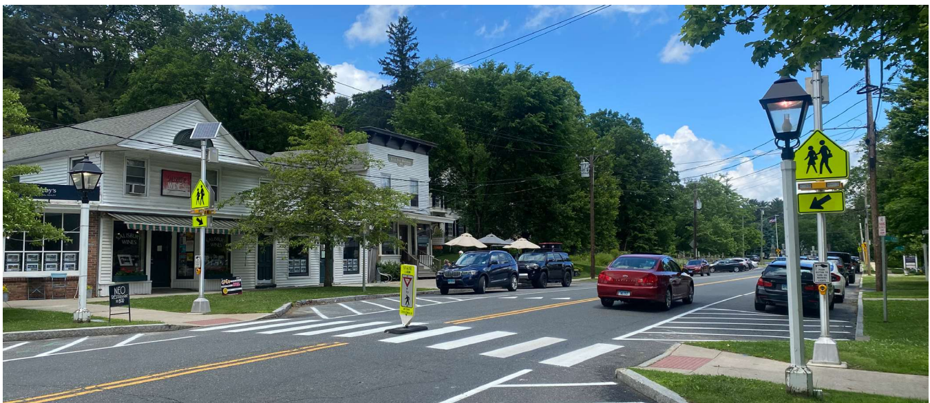
RRFB Installation, Route 44, Salisbury, CT
