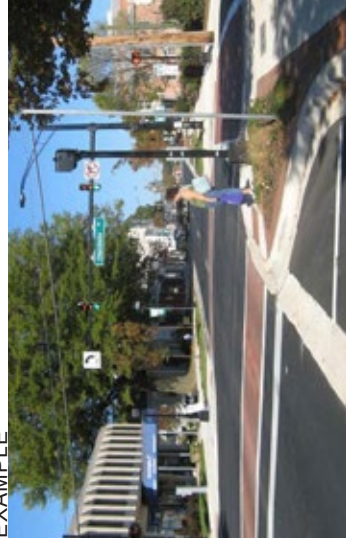
Figure 69: A curb extension reduces crossing distance
